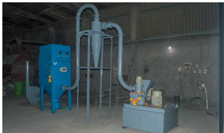
▶ Installation of DP® ACM-10 in West India for grinding of zinc metal
